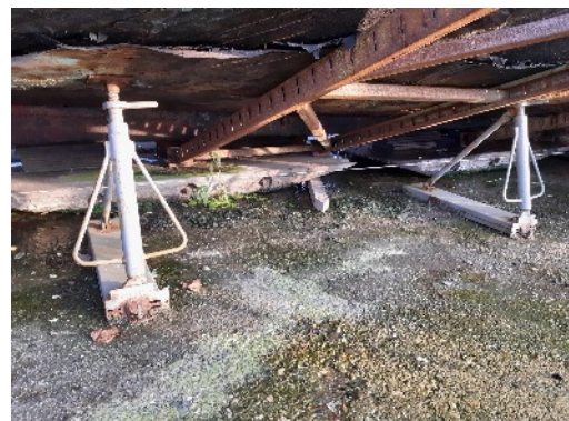
Supports under the engine room
